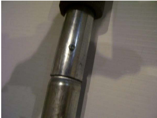
Upper (dog leg) and Straight Sections of Upright Posts joined and secured with a Screw.
